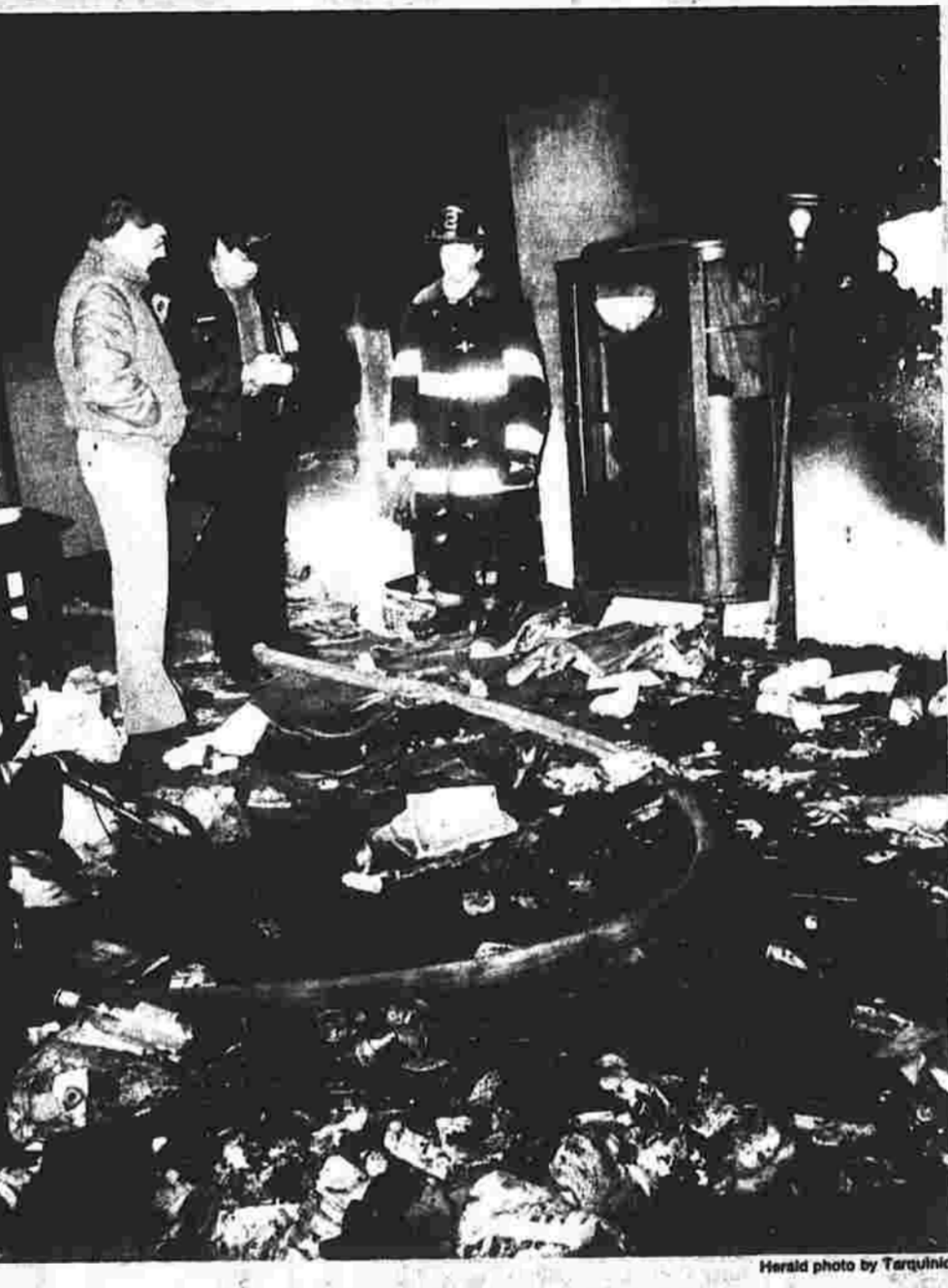
Police and fire officials inspect the damage after a fire Tuesday afternoon in an apartment at 436 North Main St. The tenant suffered burns during the blaze and was listed in critical condition at Hartford Hospital.
